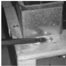
Image 1 Removing bracket from skid
